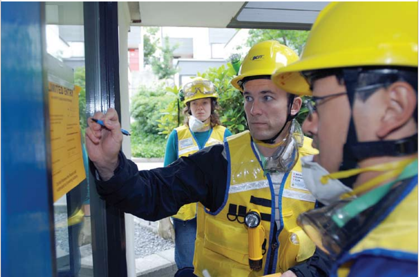
Emergency Response Team doing a Rapid Damage Building Assessment.
